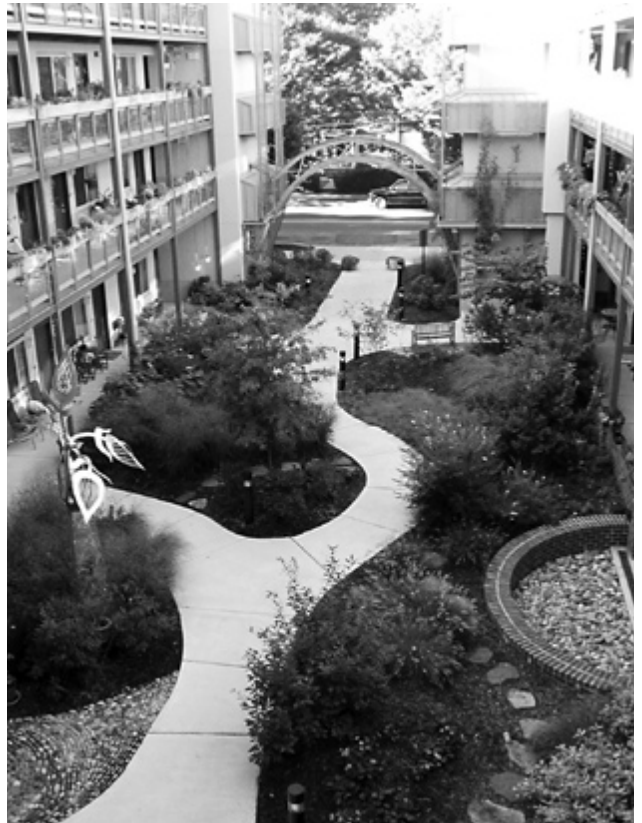
Eastern Village Cohousing in Silver Spring, MD is one of the first residential buildings in the U.S. to attain a LEED Silver rating for environmental performance.
